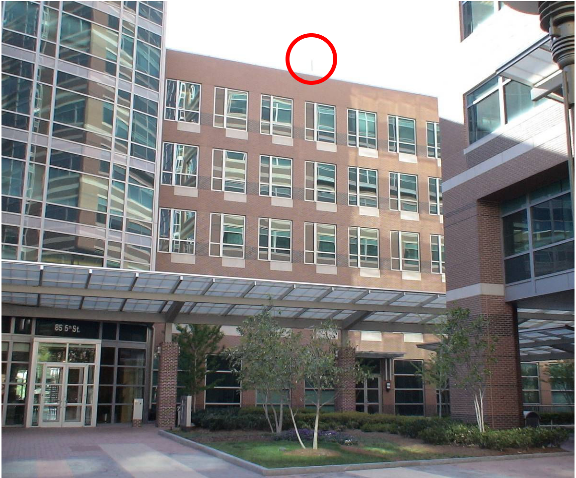
Figure 8: The Technology Square Research Building (TSRB) North AP and surrounding area. The red circle indicates the location of the transmitting antenna.
