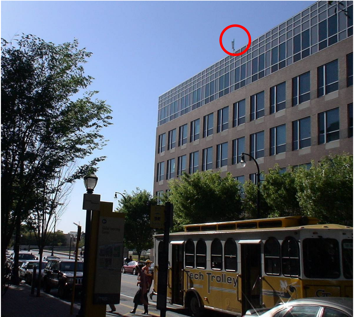
Figure 7: The Technology Square Research Building (TSRB) South AP and surrounding area. The red circle indicates the location of the transmitting antenna.
